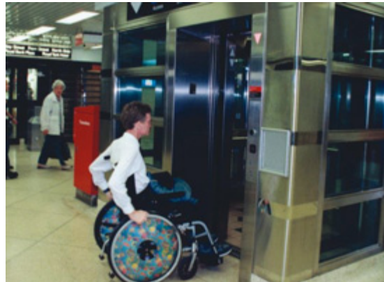
Elevators designed to TTC standards
